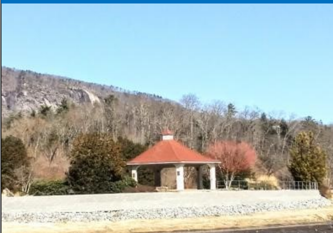
New Lake Lure Gazebo Seawall
